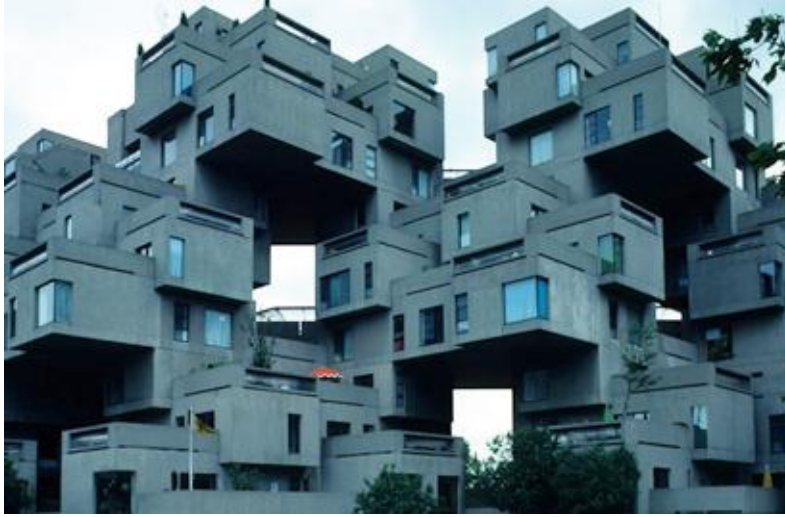
Şekil 3.30. Habitat Konut Grubu, 1967, Montrel, Canada - Moshe Safdie ( http://www.greatbuildings.com/buildings/Habitat_67.html , 2012)
