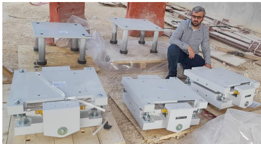
Figure 2.18. Spherical Bearings before Installation.
