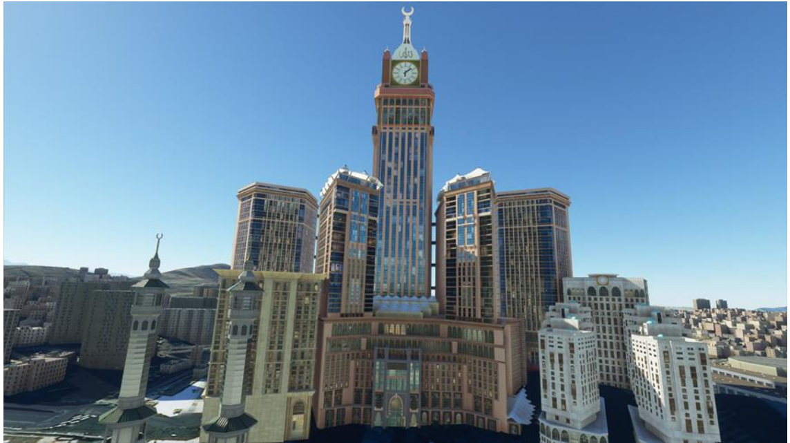
Figure 1.2. Makkah Clock Royal Tower, 601 m height mainly constructed from concrete.
