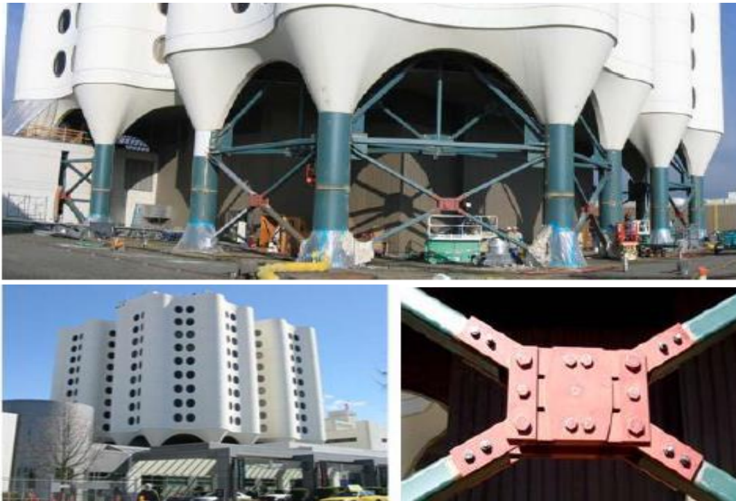
Figure 2.19 General View of St. Joseph medical center patient tower with PFDs (Shao et al., 2006).
