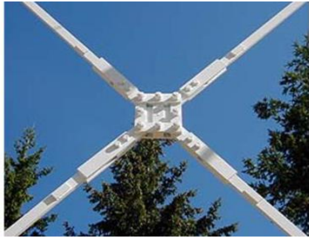
Figure 2.15 The use of PFDs in Provincial Police Headquarters in Quebec, Montreal, Canada (Pall and Pall, 2004).
