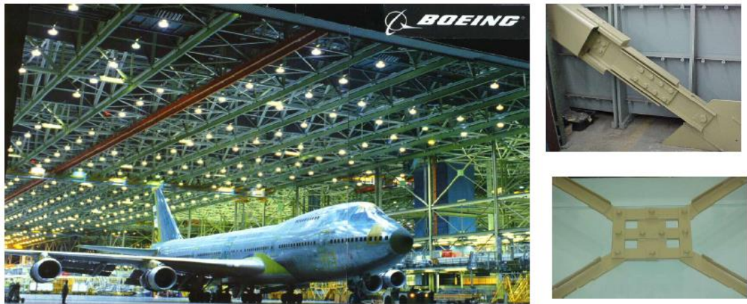
Figure 2.12 Improving the seismic resistance of the boeing commercial airplane factory by PFDs, everett, washington, USA (Pall and Pall, 2004).
