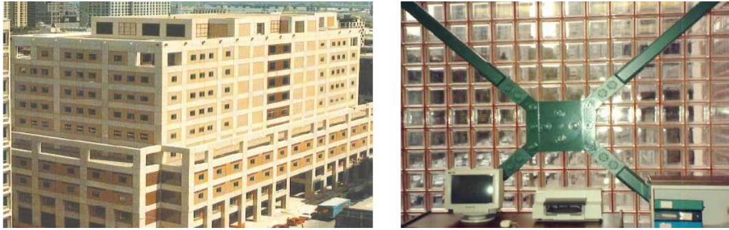
Figure 2.17 Concordia University Library Building with the addition of PFDs, Montreal, Canada (Pall and Pall, 2004).
