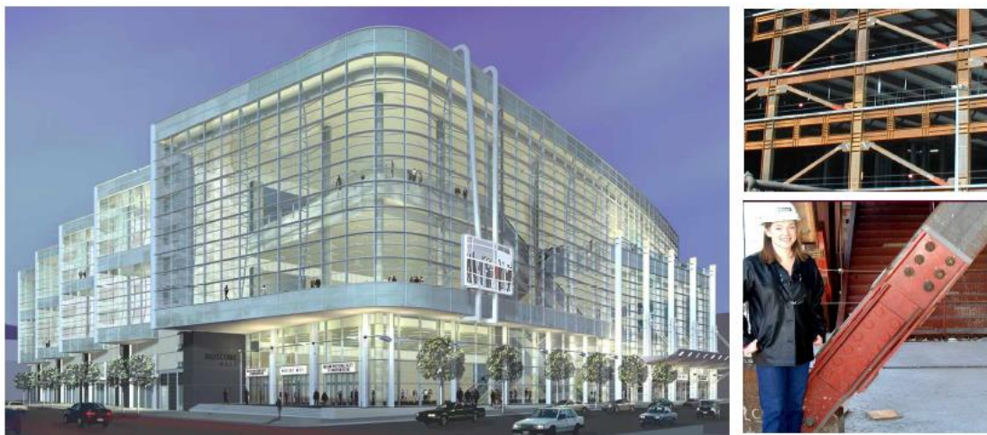
Figure 2.13 Moscone west convention center equipped with PFDs, San Francisco, USA (Pall and Pall, 2004).
