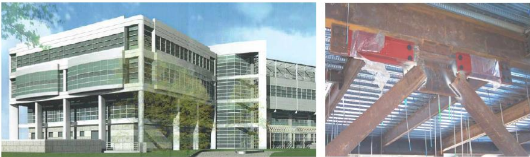
Figure 2.18 A view of Sharp Memorial Hospital's ambulatory care center with PFDs, San Diego, California, USAResponse (Pall and Pall, 2004).
