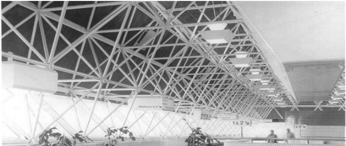
Figure 8. The Nodus space frame, Gatwick railway station
