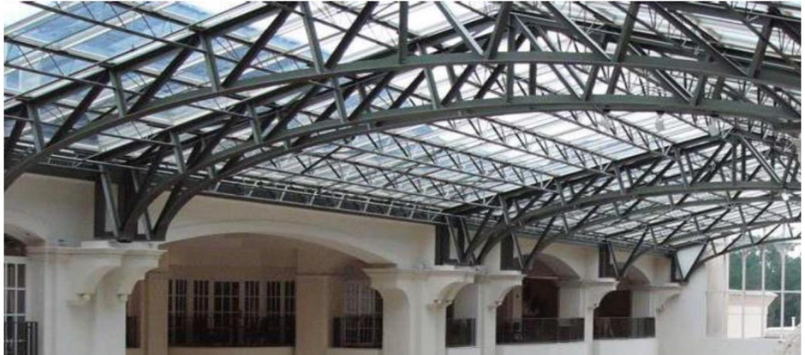
Figure 10. The Barrel vaults
