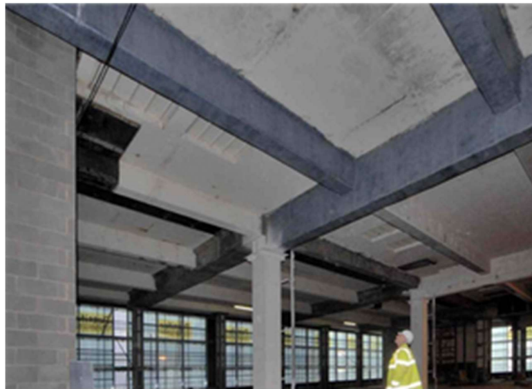
Figure 1.10. The strengthened beams by using CFRP.
