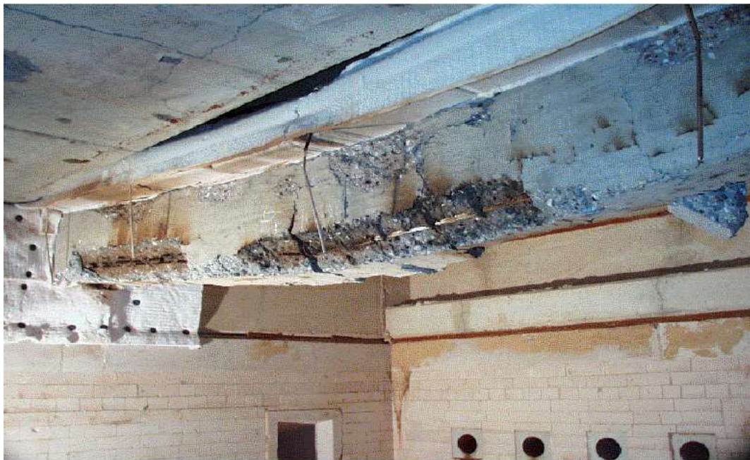
Figure 1.4. The effect of overloading (Muneeb, 2015)
