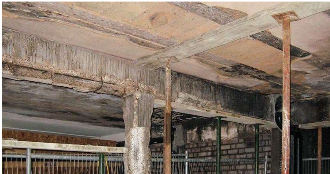
Figure 1.2. The effect of fire on RC elements (Emmons 1994).
