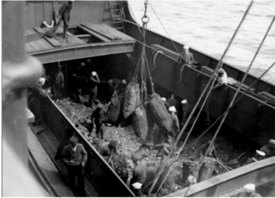
Figure 5.3: Coaling the H.M.C.S. Niobe from a lighter or barge alongside c.1910-1914. George Metcalf Archival Collection, Canadian War Museum, 20090174-011.
