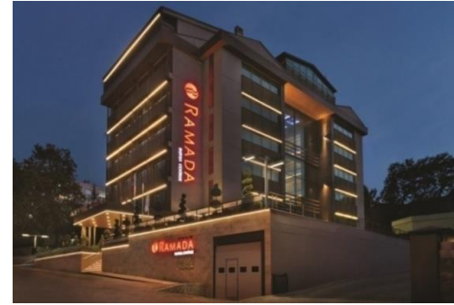
47 Ramada Bursa Çekirge Otel / Hera Termal & SPA
