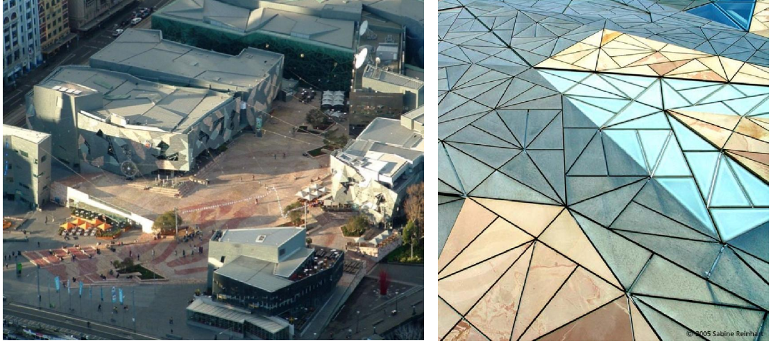
Şekil 5.22. Federasyon Meydanı, LAB Architecture Studio + Bates Smart, Melbourne, 1997-2002 ( http://www.fedsquare.com )
