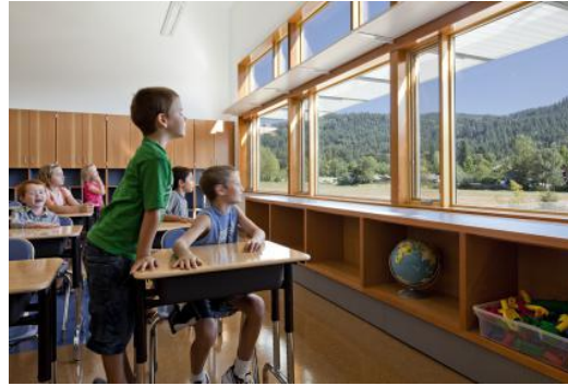
Şekil 2.14. Thurston Elementary School, ışık rafı kullanımı ( http://archive.2030palette.org/swatches/view/intermediate-light-shelves/thurston_elementary_school_springfield_public_schools_1.jpg , 2019)
