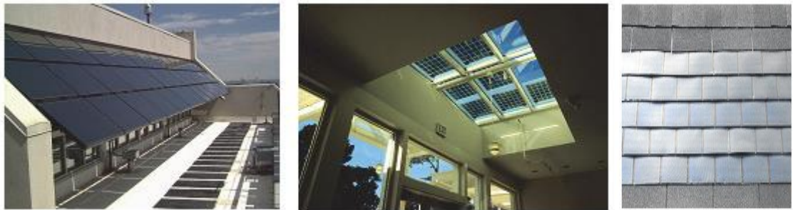
Figure 3.7. Examples of BIPVs developed by the NREL (Lawrence et al. 2013)
