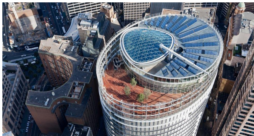
Figure 3.6. PV panels on the roof of 1 Bligh Street, Sydney (CTBUH's Database 2017)
