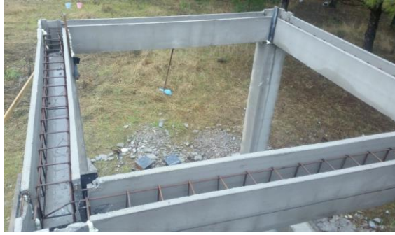
Figure 3.5. Formwork installation of columns and beams.
